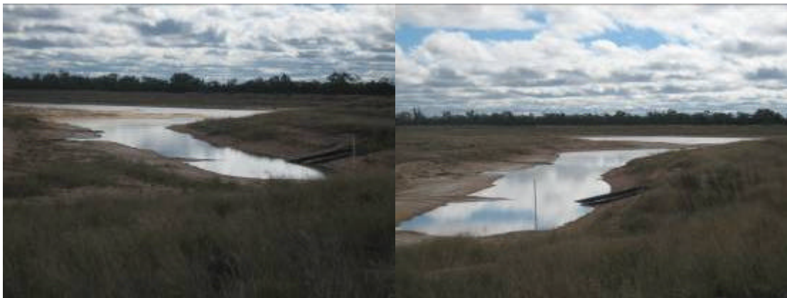
Photo Taken 18/06/08. P5 & P6 Dam. The stick to the right in picture is the capacity measure.
